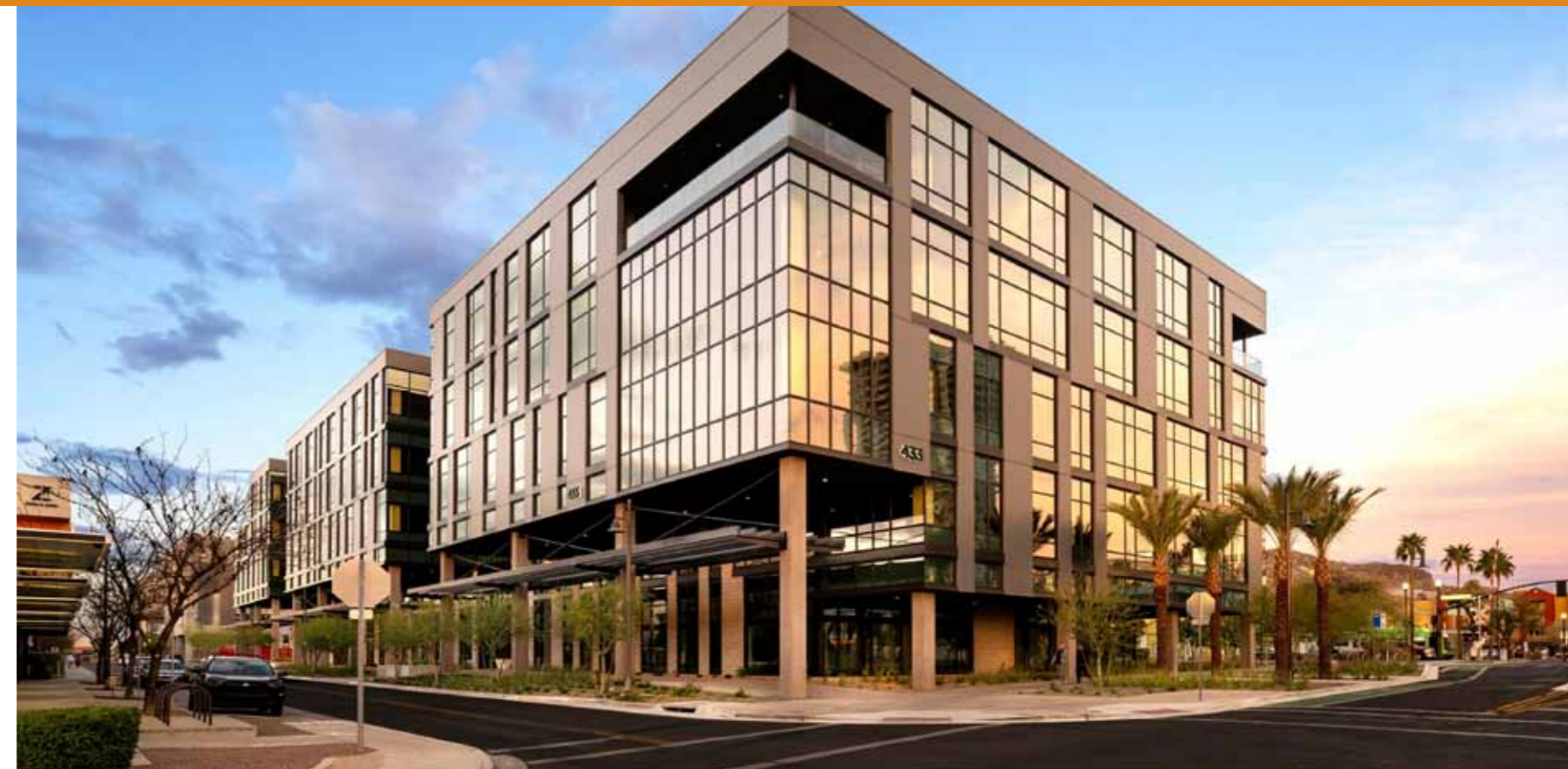
Beam on Farmer, Phoenix, Arizona, USA / Skyline Facades
